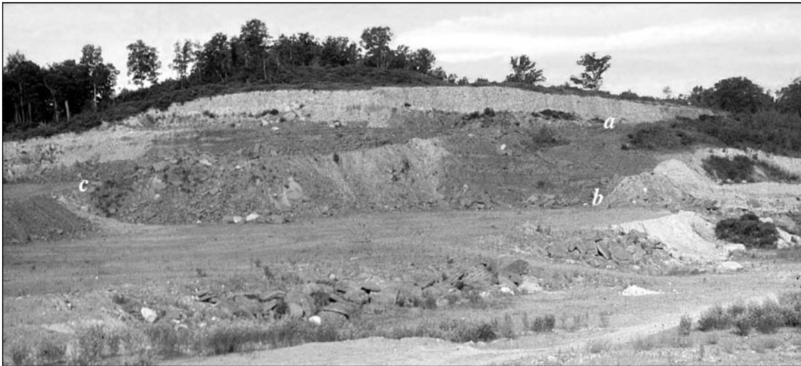
Figure 55. Riker Hill Quarry (Stop 7) ca. 1969: a, contact between Hook Mountain Basalt (above) and Towaco Formation (type section); b, top of gray bed, unit 6; c, base of gray bed unit 15-16 (Figure 56).
